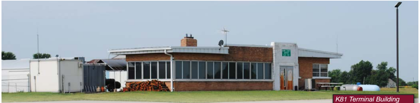
K81 Terminal Building Image Source: Lochner.
